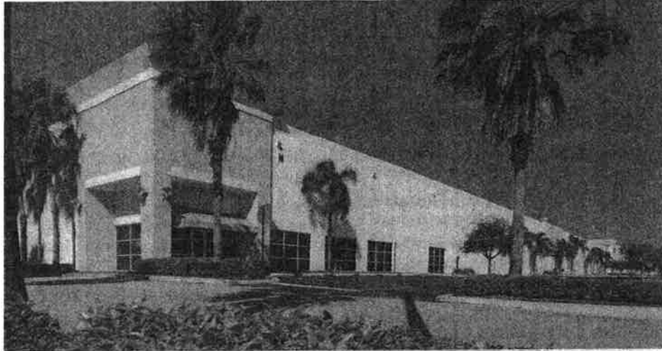
TA Products LLC leased 93,700 square feet at Seneca Industrial Park.
